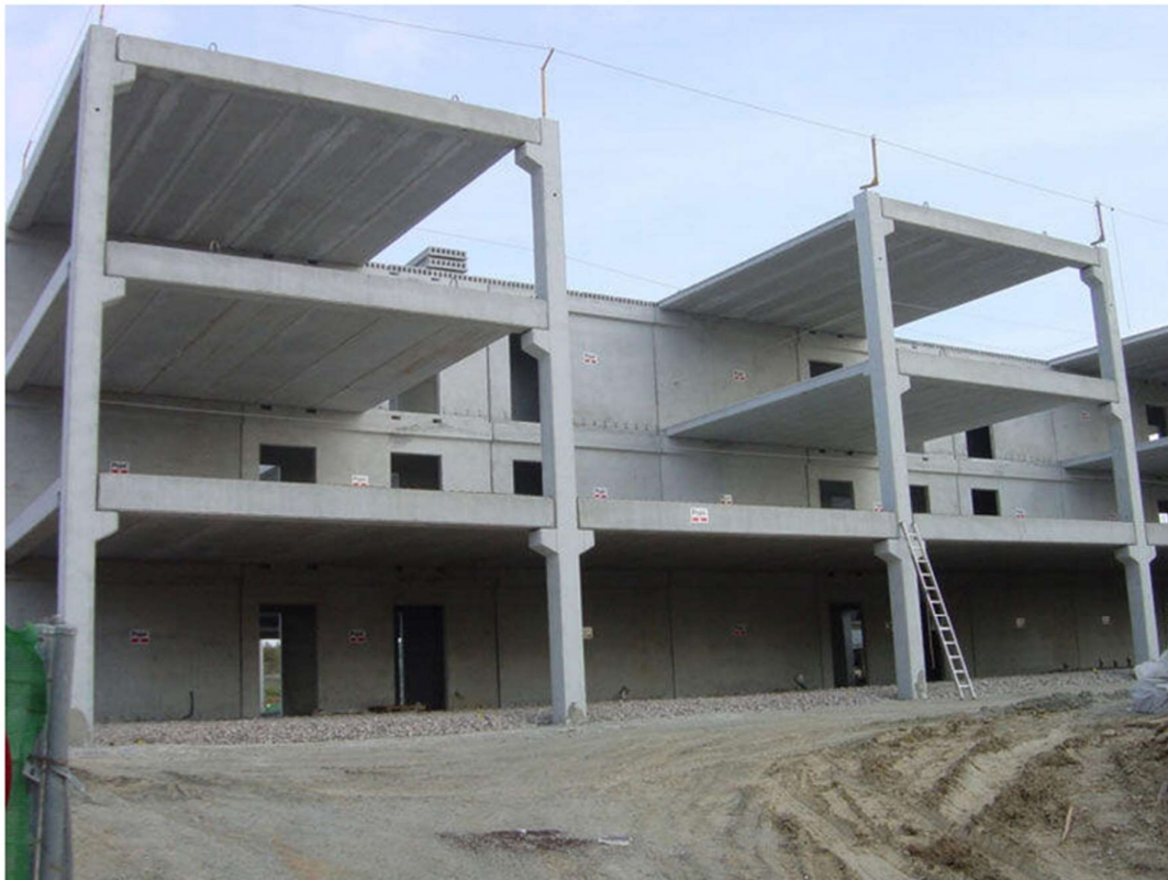
Corbels in precast construction
